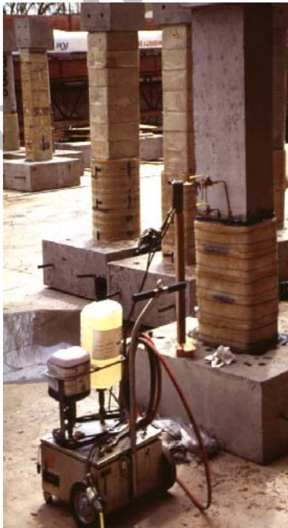
Fig. 6. Wrapping of FRP straps around columns and pressurizing for active confinement.
