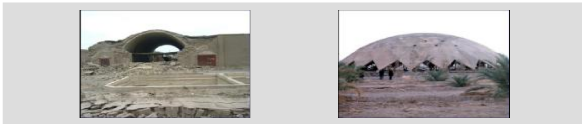
Figure 6- The effect of a geometrical form of the building on its stability, the right picture: a fair hall with the ceiling of space structure and a one-layer coating in newly repaired Arge Bam. The left picture: a mill building with annular barrel vault with a span of 10 meters.
